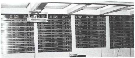
Earth station identification board provides Communications Center operators with, from left to right, station number, alphabetical listing, double-letter code, country in which located, computer designation, automatic acquisition code letters, and message transmission teletypewriter machine identification. Small panel at upper left of picture alerts duty operators to incoming messages by means of blinking lights.
