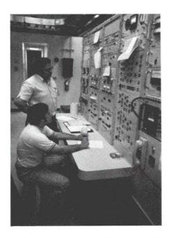
Roger Miner (standing), was the chief station engineer with an AM broadcast station prior to joining the Southbury staff. He and Dave Davies discuss the performance of the station's monitoring equipment used in pointing the 42-foot full performance antenna.
