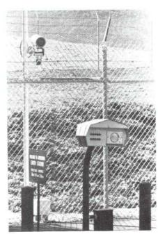
the visitor is to be admitted, the gate is operated remotely from either of the control units in the building. The gate closes automatically once the vehicle has passed through. During normal working hours, Monday through Friday, the gate is controlled from the console in the Administrative office. During the remaining time, control is performed by the operations personnel on duty in the Control Room.
