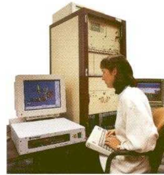
The frame relay access switch offers an International Telecommunication Union-Telecommunications Sector (ITU-T) standards-compatible interface that can be used to interconnect any number of LANs, workstations, and personal computers over the ACTS system.
